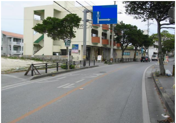
Example of constructing a discontinuous guard fence on an uninterrupted straight road; In some cases; accidents were not reduced
